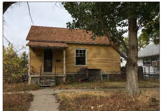
c1912 Hall-and-Parlor dwelling, 228 E. 8 th St.
