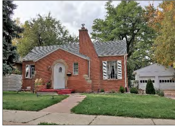
c1936 Tudor Revival dwelling, 1636 S. Spruce St.
