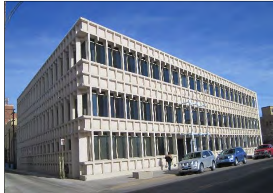
1961 International Style building, 100 West Midwest Ave.
