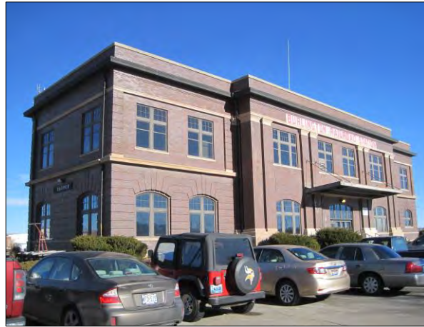
1916 Chicago, Burlington & Quincy Depot, 360 N. Wolcott St.
