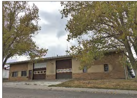
Casper Fire Station No. 6, 280 Valley Dr.
